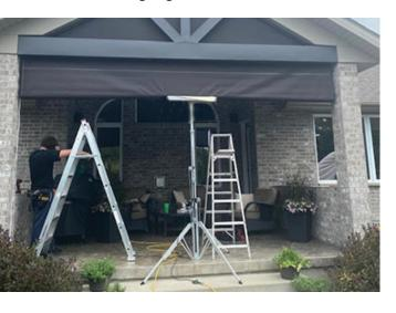
**LIFTEASY** has a solid telescopic mast made out of aluminum alloy that has a built-in level to ensure stability in all situations.
